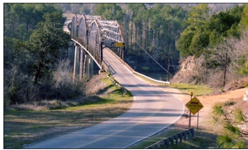
The Old Steel Frame Bridge at Claiborne, Alabama.
