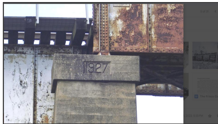
Date Stamp, 1927, on the Top of a Column, Atmore Rail Overpass.
