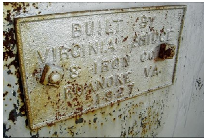
Date Plate on Atmore Rail Overpass
