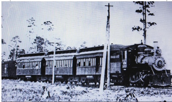
Early Gulf, Florida, and Alabama Corporation (GF&A) Train Approaching McCullough.
