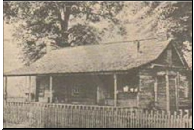
This House was either taken from Fort Crawford and moved a short distance away or built of materials taken from structures at Fort Crawford. It survived into the 20th century.
