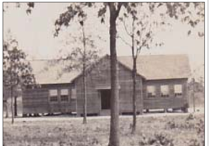
Elementary School at Alaflora
