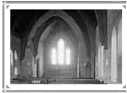
Interior View toward Chancel, from 1934
